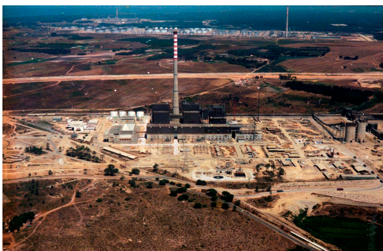
Figure 9. Thermoelectric plant (foreground) and refinery (background) under construction in the Municipality of Sines, Portugal (1970s)
