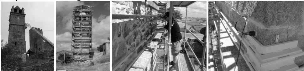
Figure 2: Measurements before and after the rehabilitation showing also some sensor locations
