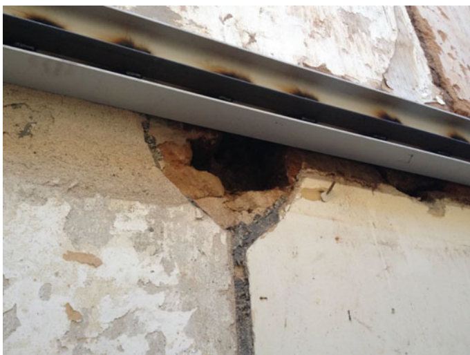
Fig. 3 Metal beam and facade containment
