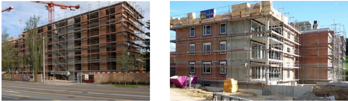
Figure 1. Examples of low- and mid-rise URM building construction [2]
