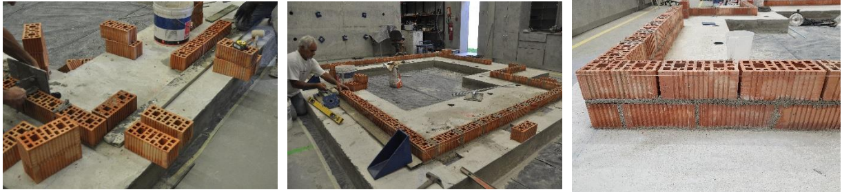
Figure 6. Construction of the URM walls
