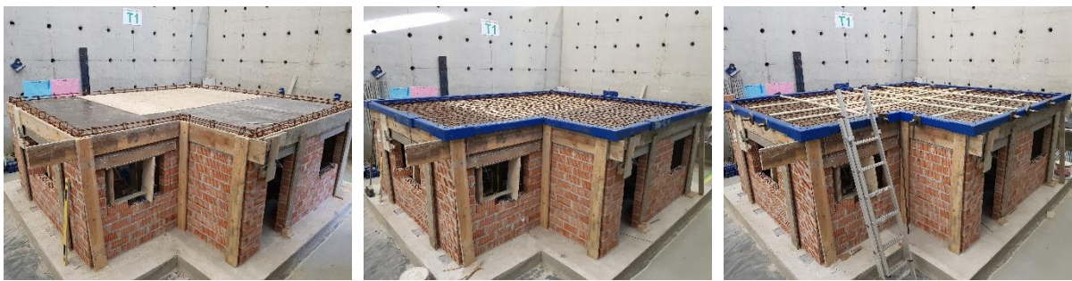
Figure 7. Construction progress of the RC slab
