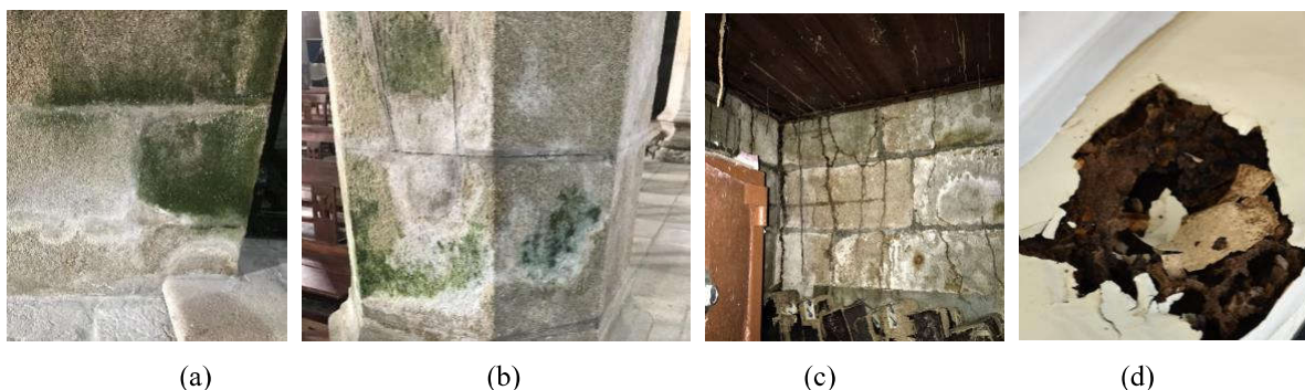
Figure 4: Algae observed on (a) interior walls and (b) column base; (c) termite infestation behind altar; (d) rot in altar
