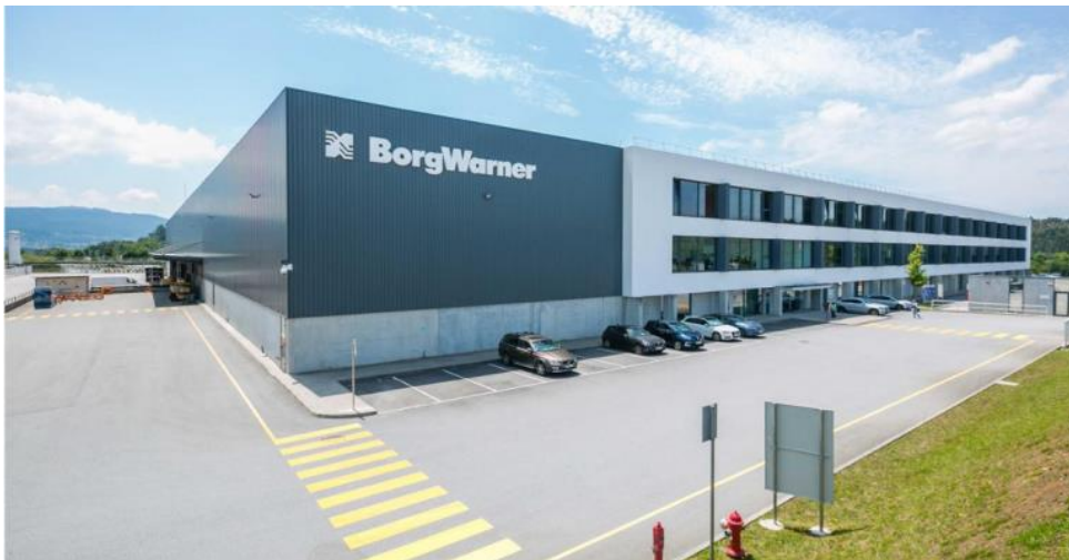
Figura 5 – Fachada da BorgWarner Emissions, Thermal and Turbo Systems – Viana do Castelo
