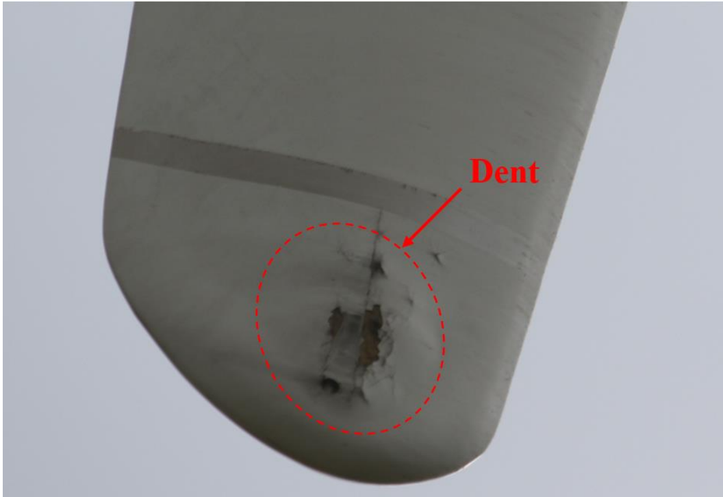
Figure 2.12: Dent in a WTB detectable via visual inspection. Source: [29]
