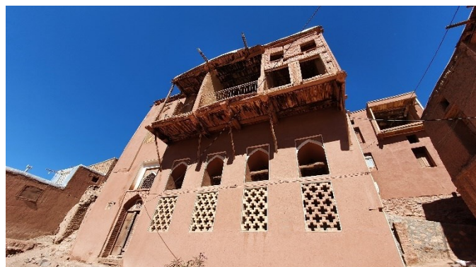
Figure 99 :Net bricks on the façade of the buildings in Abyaneh, by author
