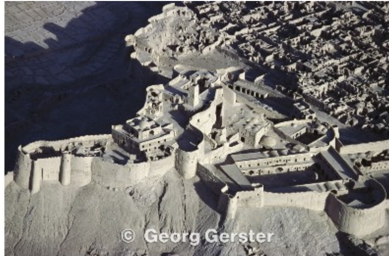
Figure 29: largest adobe building(citadel) in the world-Bam, Iran, it was a large fortified with a citadel that was almost completely destroyed by an earthquake in 2003. By Georg Gerster,1977
