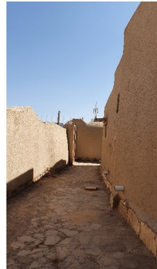
Figure 140 :Harmonious architecture inside historical part of village, by author
