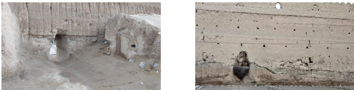
Figure 165: New entrances in the walls of the fort, By author
