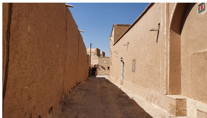
Figure 139: similar walls of the buildings without windows, by author
