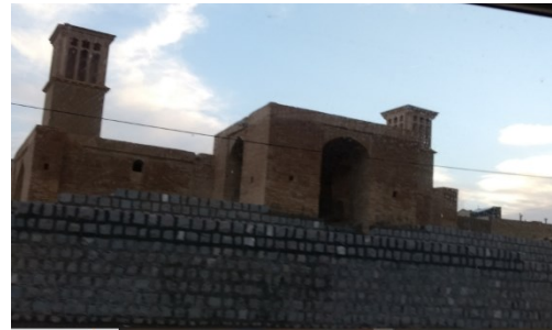
Figure 192 :water reservoir, outside the fort
