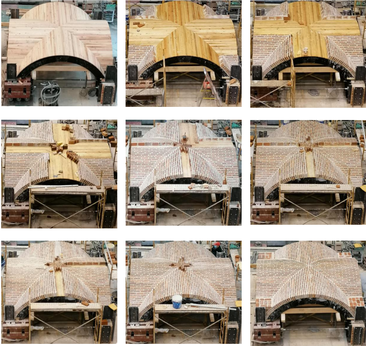
Figure 5-7. Construction sequence of the unstrengthened specimen.
