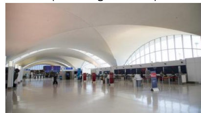
Air Terminal, St. Louis (1954)
