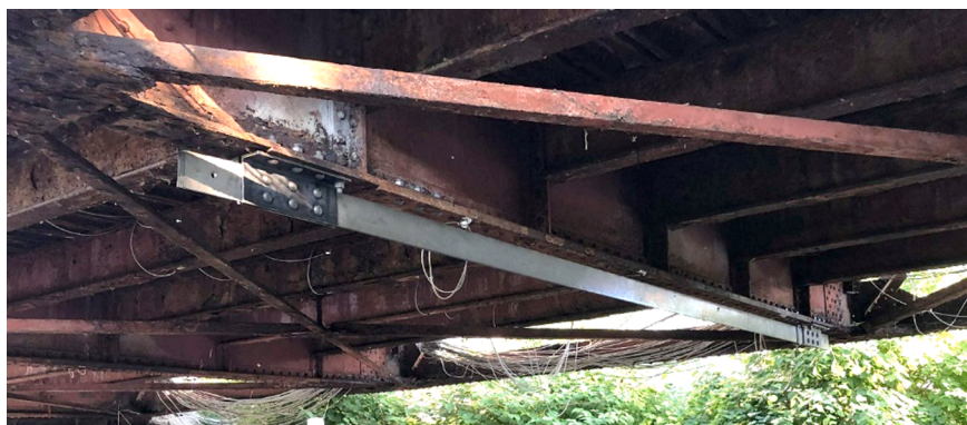
Fig. 19. Final configuration of SMA-strengthened girder in Petrov Bridge.
