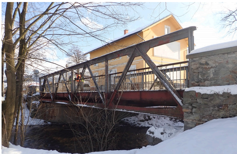
Fig. 2. Historic steel road bridge in Petrov nad Desnou, Czech Republic.
