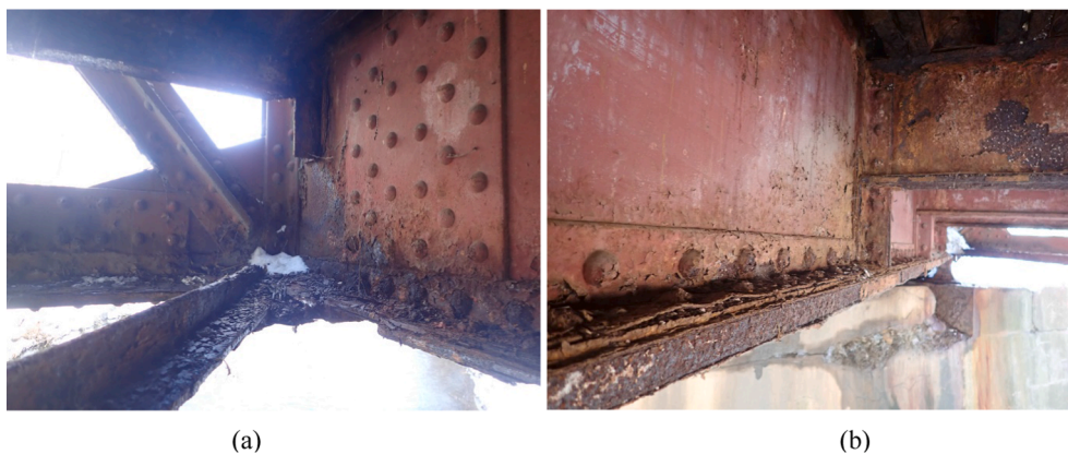
Fig. 3. a) Lower chord joint and b) lower flange of cross-beam.
