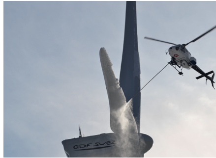
Figure 2.15 – Ice removal with hot water sprayed from the helicopter [24].
