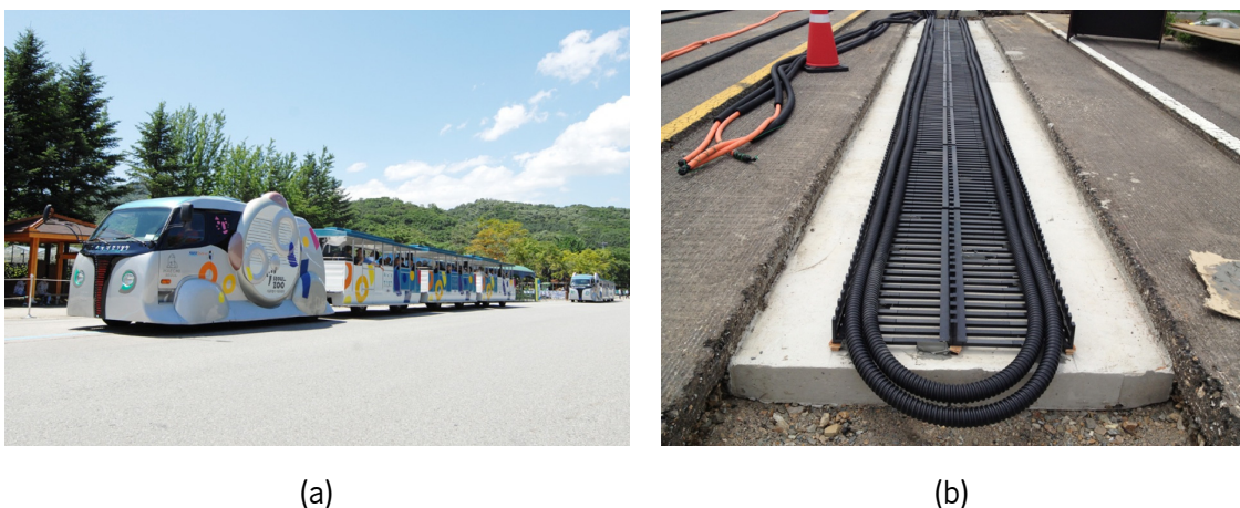
Figure 99: (a) OLEV tram in Seoul and (b) system's primary coil during the installation phase. Source: [107].
