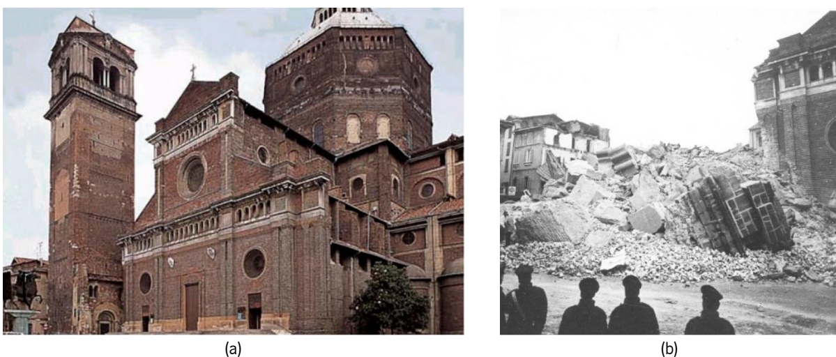
Figure 7.1. Civic Tower of Pavia, Italy: (a) tower and cathedral before the collapse; (b) ruins after the collapse. Images from Binda et al. (2007), Anzani et al. (2009).
