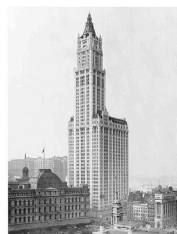
(3) Woolworth Building (Manhattan, Nova Iorque)
