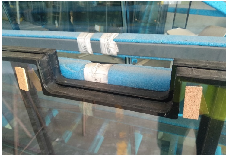
Figure 2.6. Glazing with the detail that allows for the introduction of the locking mechanism.
