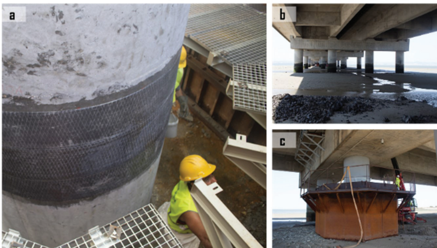
Fig. 4: Strengthening of bridge piers, Vasco da Gama Bridge (from Reference 68)
