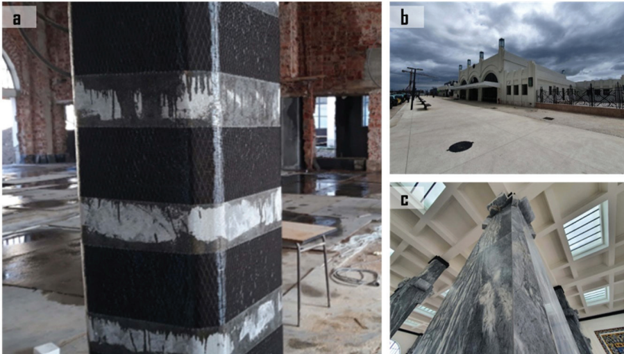
Fig. 2: CFRP jacketing of columns on Estação Fluvial Sul e Sueste: (a) jacketing on RC columns; (b) the fluvial station; and (c) finished strengthening of columns (from Reference 66)
