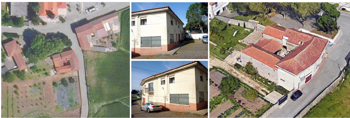
Figure 38 - Project location and outside view
