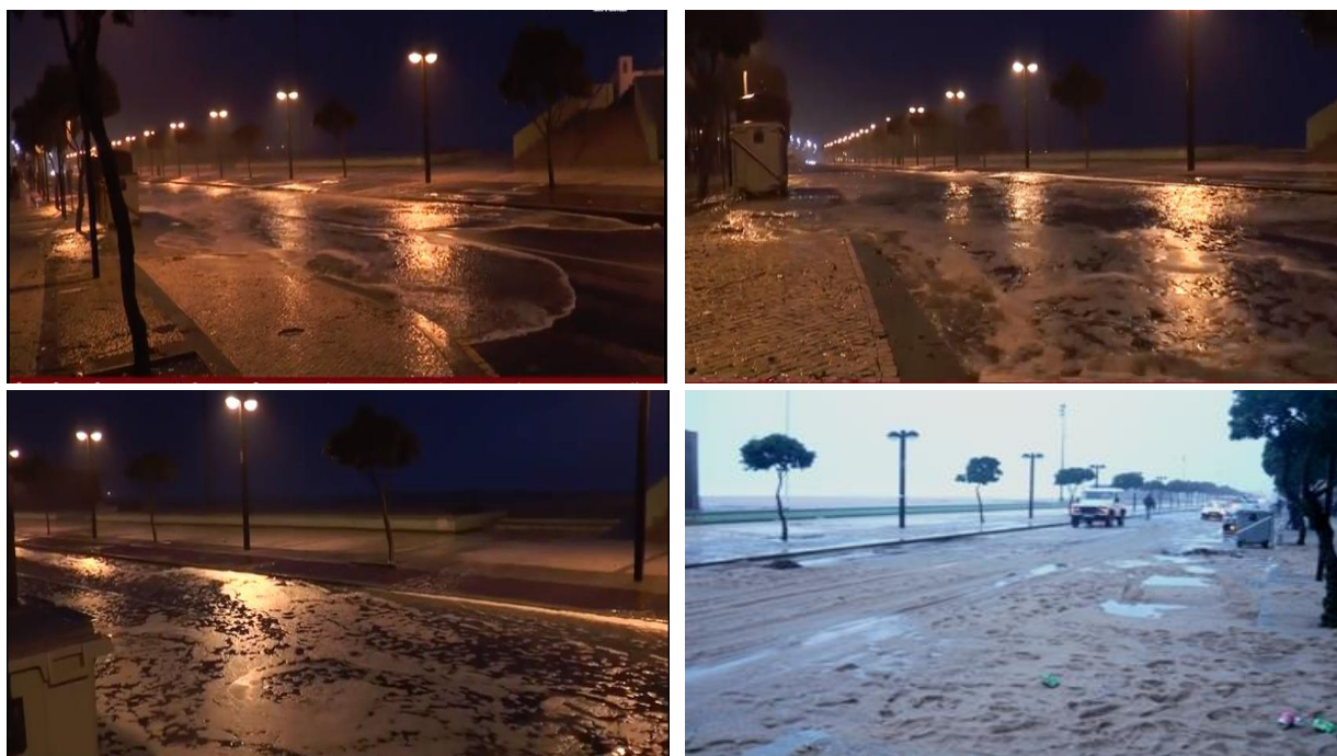
Figure 1.5: Flooding events in the city of Póvoa de Varzim – storm of 2014 (Vieira, 2014).
