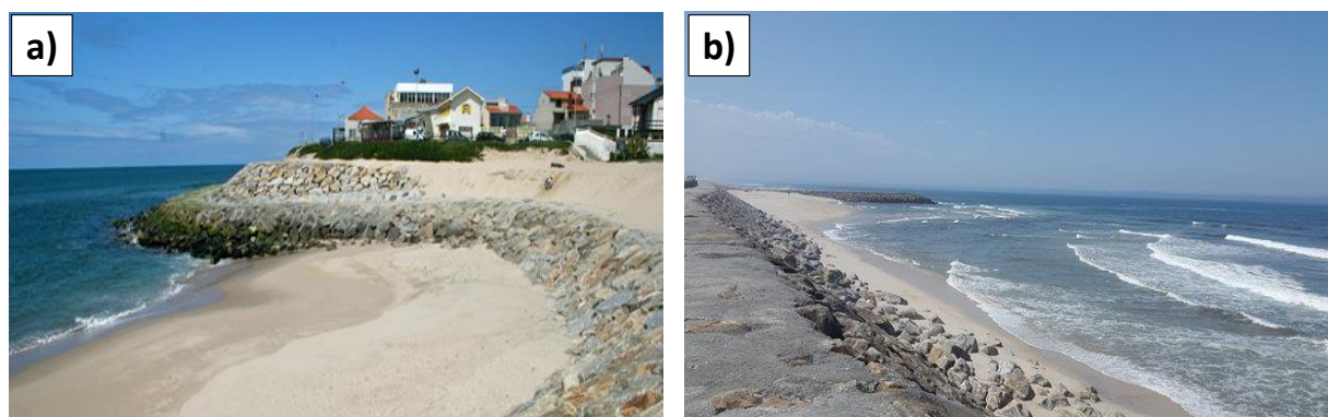
Figure 2.24: Longitudinal revetments at Ovar coast, Portugal: a) Cortegaça; and b) Furadouro.
