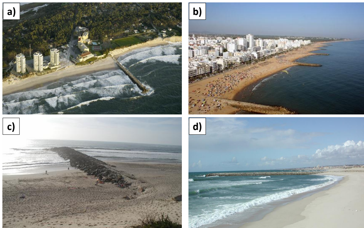
Figure 2.22: Groins in Portugal: a) Ofir; b) Lagos; c) Madeira; and d) Espinho (Vieira, 2014).
