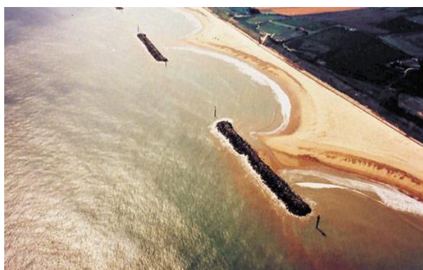
Figure 2.15: Formation of tombolo in the leeward side of an emerged breakwater due to diffraction currents (Vieira, 2014).
