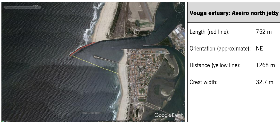
Figure 5.5: Vouga estuary: Aveiro north jetty characteristics (2018).
