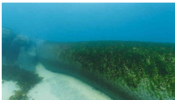
Figure 2.45: Type of organic growth associated with geotextiles (Shin and Oh, 2007; Vieira, 2014).
