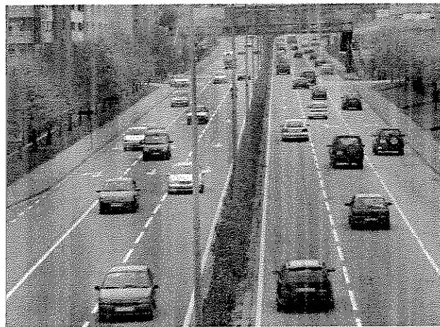
Photograph 3 – Urban road of high traffic capacity
