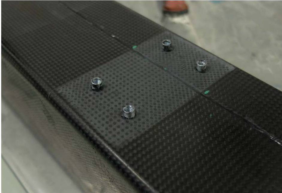
Figure 5.20 - Treated area of final composite shell area used to attach the steel bearing component
