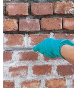
Finishing mortared joints pointed with Mape-Antique MC
