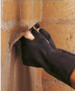
Application of the first layer of Planitop HDM Maxi
