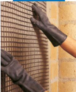
Positioning of Mapegrid G 220
