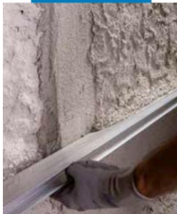
Levelling the surface of Mape-Antique MC with a straight edge
