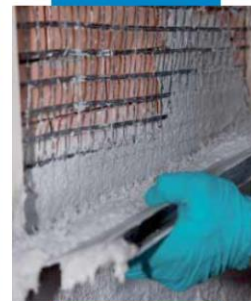
Application of Planitop HDM Restauro system with Mapegrid G 220 on a brick wall
