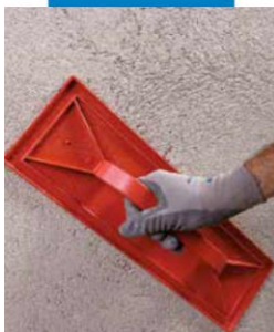
Levelling the surface of Mape-Antique MC
