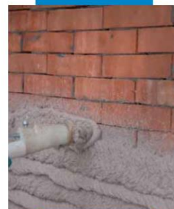
Application of Planitop HDM Restauro by spray on a brick wall
