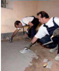
Application of the first layer of Planitop HDM Restauro by trowel on the outer face of a vaulted ceiling
