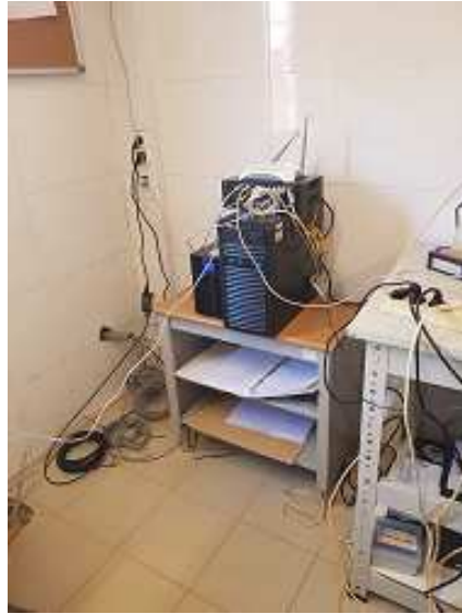
Picture #30 – Assembly and setup server, router, switch and UPS
