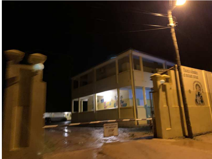
Picture #4 – HPSJB main door
