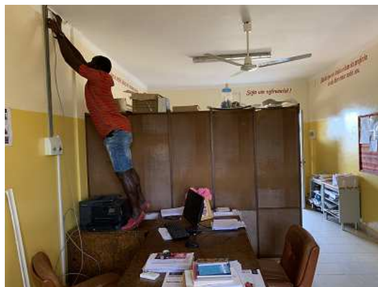
Picture #29 – Install office wired network and sockets for PC and printers
