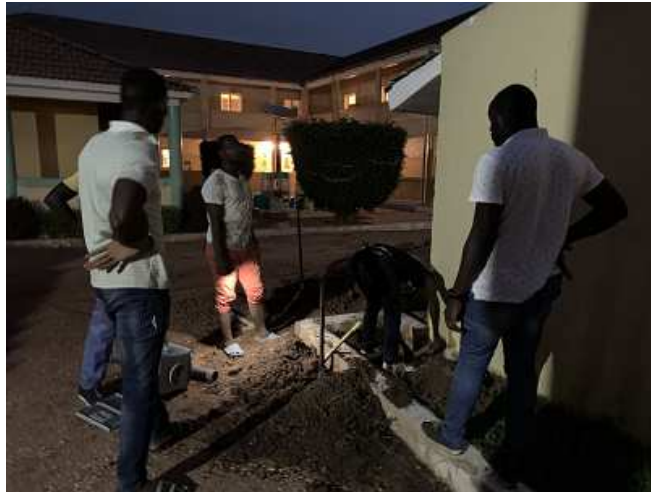
Picture #27 – Prepare wired network pipelines to cross buildings
