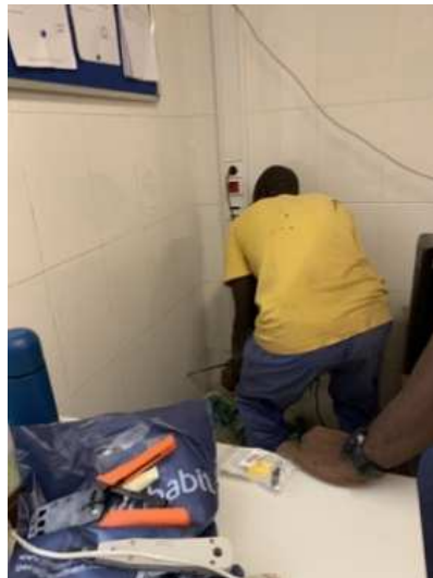
Picture #28 – Network pipelines crossing buildings
