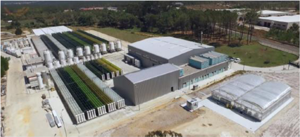
Figure 1 Aerial view of Algafarm.
