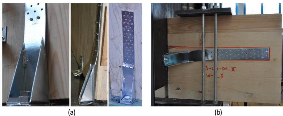
Figure 2.27 – Failure of the hold-downs loaded in tension (a) and shear (b) [37, 38].
