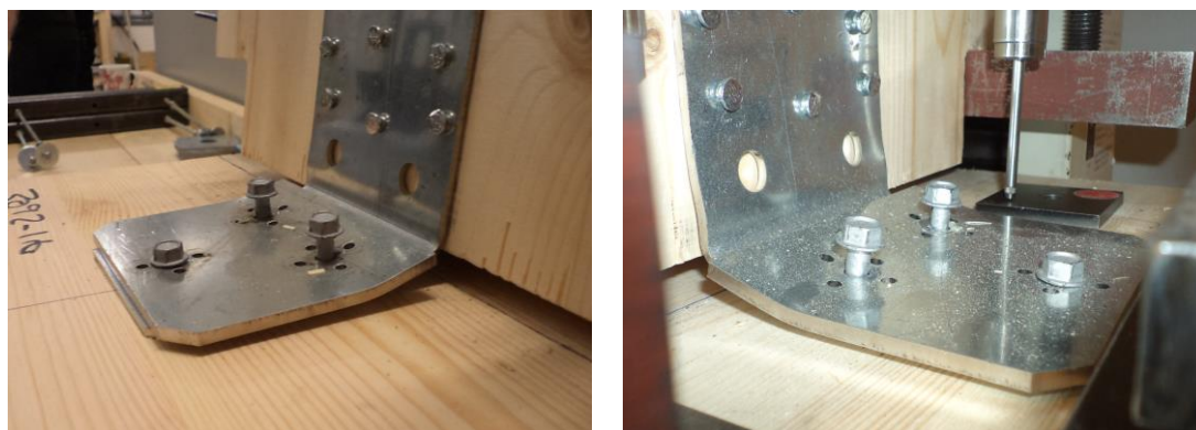
Figure 3.36 – Failure of the angle brackets AB+plate under tension loads.
