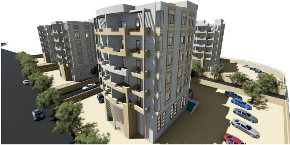
Figure 116. A general view of one of the buildings, showing the number of floors and the stores on the ground floor
