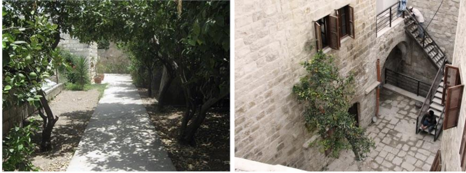
Figure 65. Vegetation used at the old city houses of Nablus to improve privacy
