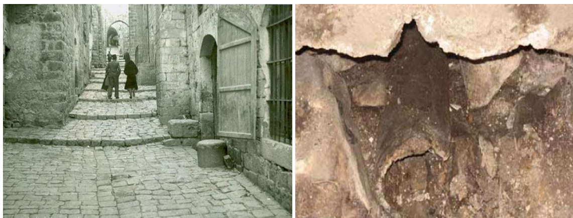
Figure 85. Street and sewers using local building materials (Palestine Remembered, n.d.)
