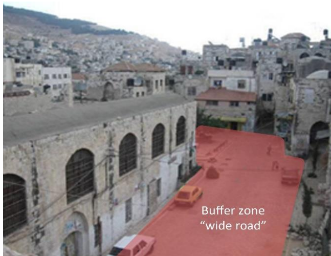
Figure 59. Applied solutions at the old city of Nablus to achieve acoustical privacy through buffer zones (Ahmad Khalaf Photography 2017)
