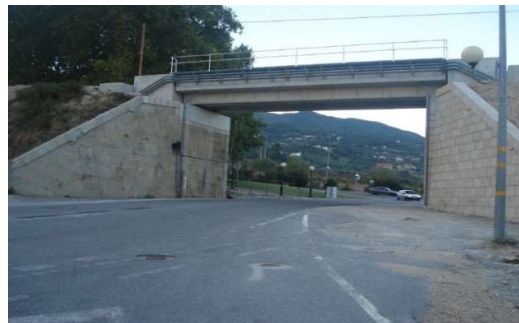
Figure 3-2 – Railway bridge view
