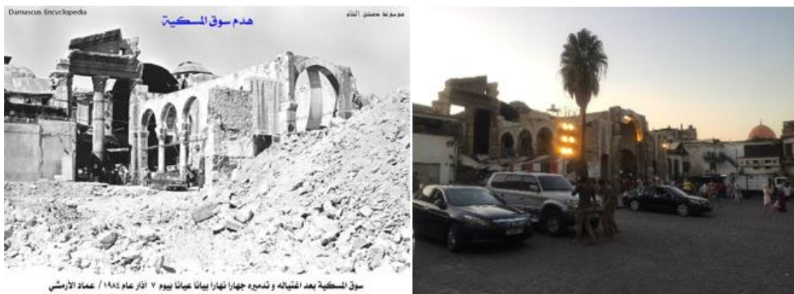
Figure 58: left: the demolition of the Meskeih market in 1984. The source: (Al-Armashi, 2014) Right: Al-Meskeih recently. The source: the author.
