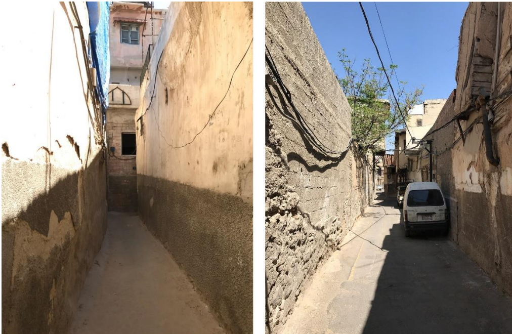
Figure 82: Photos of the thoroughfares of secondary streets. The source: the author.
