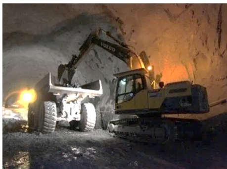
Fig.123-Carga de dumper com escombros[31]
