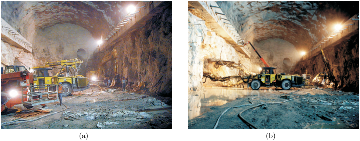
Figure 7.6: Pictures of the powerhouse complex caverns during excavation (provided by EDP).
