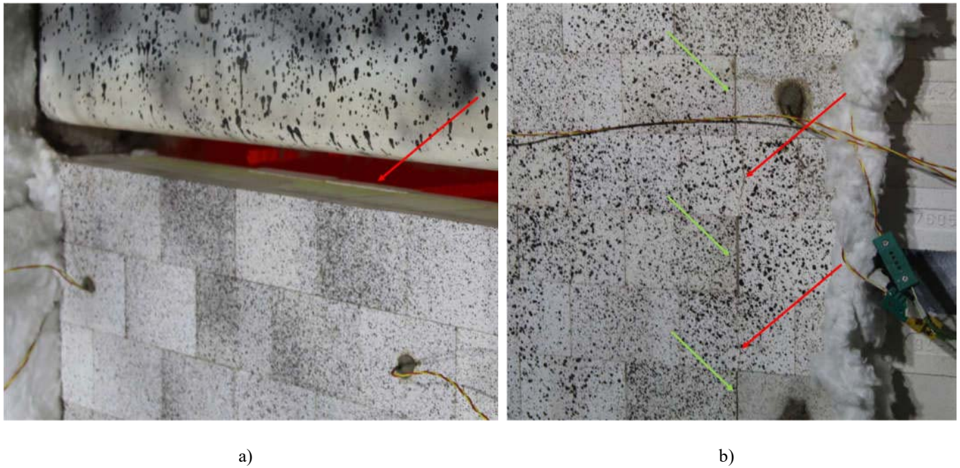
Figure 18 – Test series S03 – Damage in the wall upon completion of the test: a) Cracks in the interface between load application beam and wall (S03.HT.LL8.01), b) Vertical cracks in bricks and joints openings (S03. HT.LL8.03)
