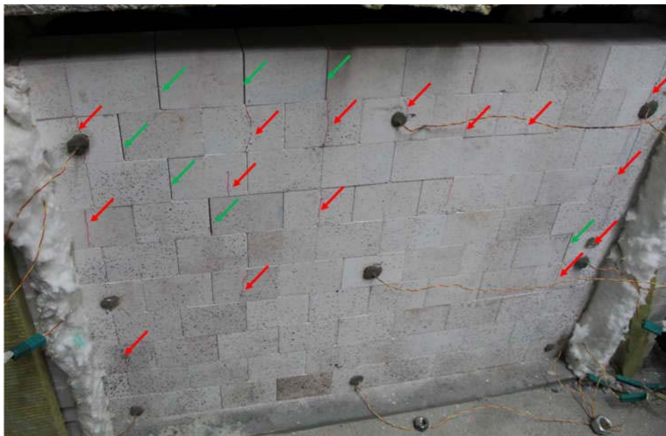
Figure 20 – Test series S04.HT.RTE – Failures in the wall: Vertical cracks in bricks and joints openings (S04.HT.RTE.02)
