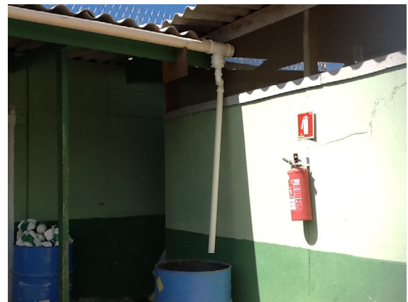
EXHIBIT 15 Collection of rainwater by the roof—site B [Color figure can be viewed at wileyonlinelibrary.com ]
