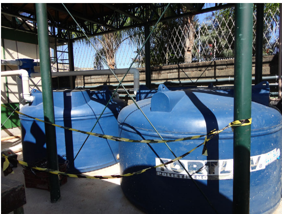
EXHIBIT 13 Tanks to reserve rainwater after treatment—site E [Color figure can be viewed at wileyonlinelibrary.com ]
