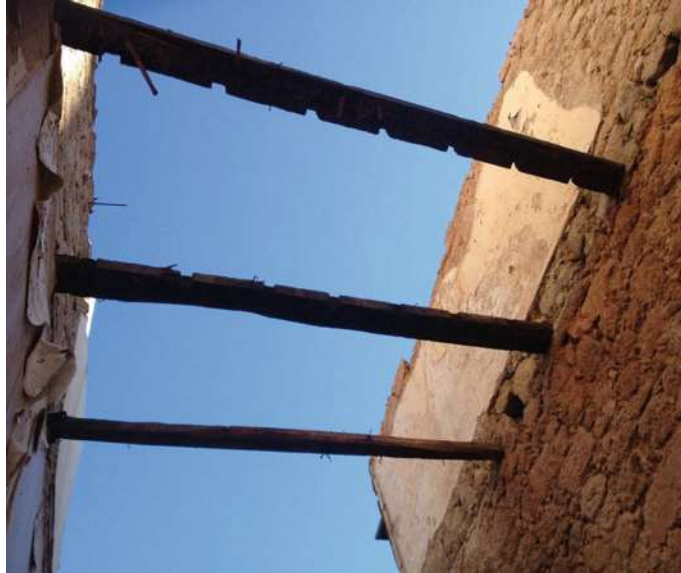
Fig. 2 Containment of facades with two existing beams
