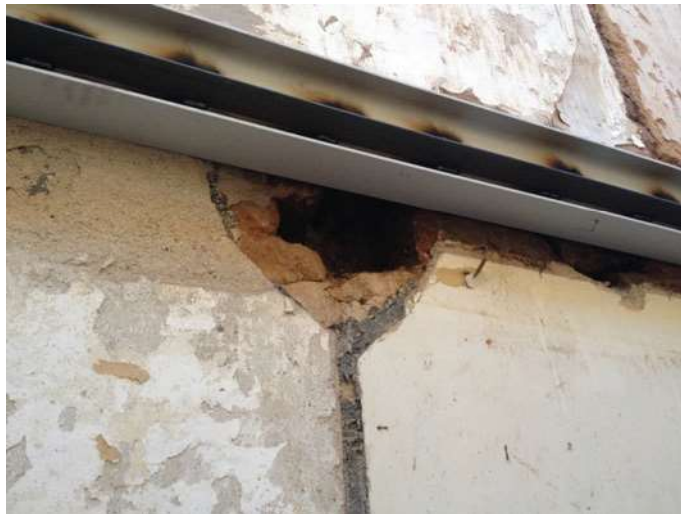
Fig. 3 Metal beam and facade containment
