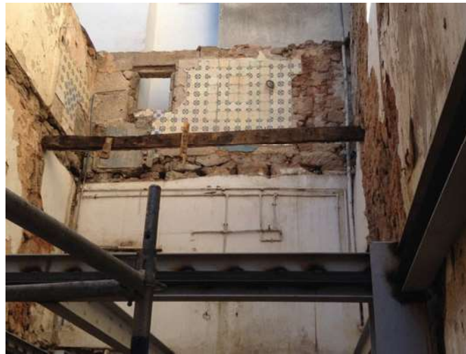
Fig. 1 General appearance of the interior of the building after demolition of its interior
