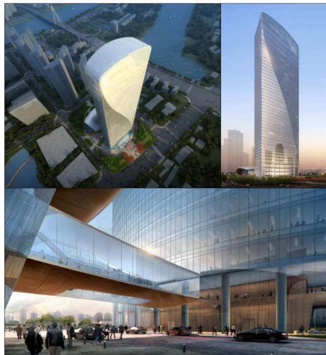
Figura 2.17— Qintai International Tower (Adrian Smith + Gordon Gill Architecture, 2012).
