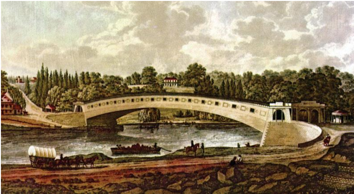
Figura 9 – Ponte de madeira "Colossus of Fairmount". Fonte: https://en.wikipedia.org/wiki/Colossus_Bridge#/media/File:Upper_Ferry_Bridge_(cropped).jpg
