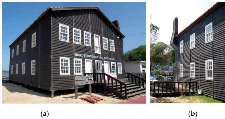
Figure 6. External views of the case study: (a) west and north façades; (b) south façade.
