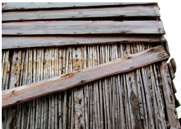
Figure 2. Reeds used as a thermal insulation layer of a timber wall (Leirosa, Figueira da Foz).
