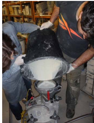
Figure 6 – (a) Wallet final aspect before grouting; (b) Introduction of grout in the pressure pot; (c) Injection of the walls
