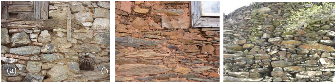
Figure 1 – Schist masonry walls: (a) and (b) with mortar joints; (c) with dry joints
