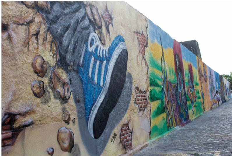
Figure 3: Rua Barbosa Lima St., n. 81. Protected set in Bairro do Recife, after the intervention (9/9/2018). Detail with approximation
