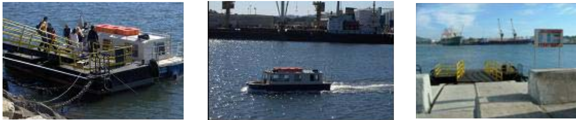
Fig. 9 –Ferryboat and its infrastructure
