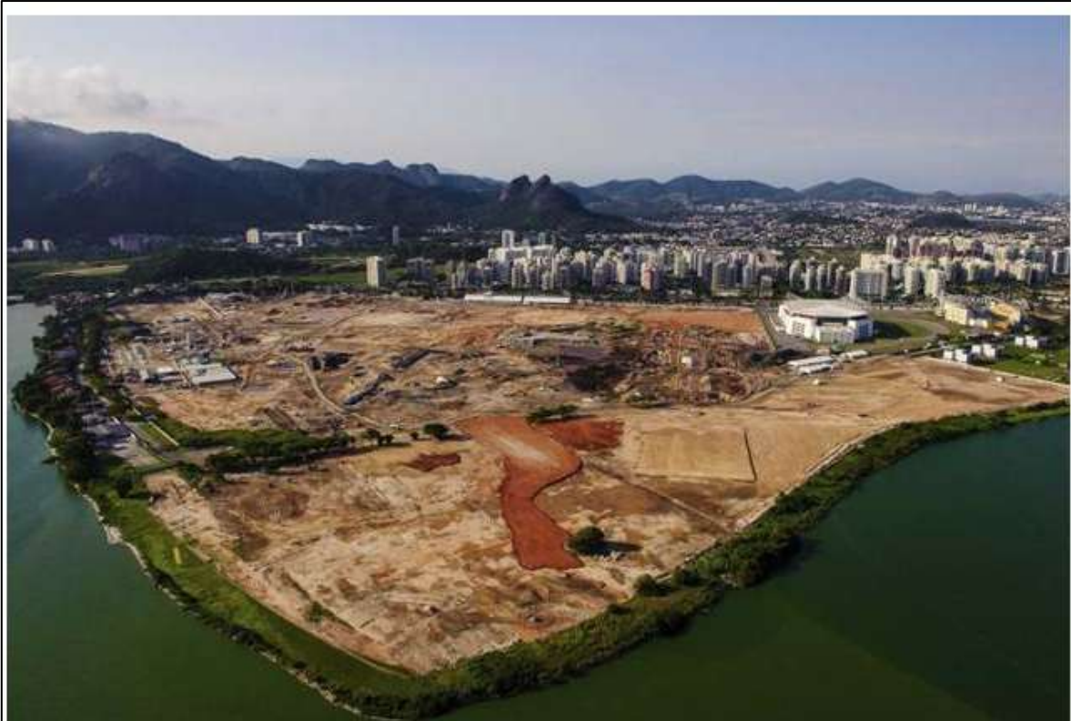
Olympic park before construction
