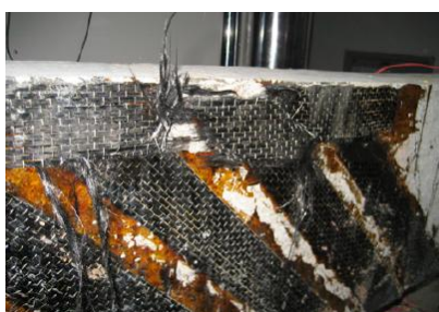
SR3/SR4 - Rotura do CFRP na face lateral superior
