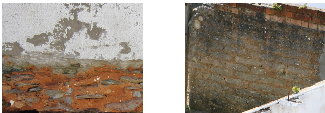
Figure 1. Materials used in Ovar's constructions. (left) mix of stone gravel and clay wall; (right) adobe wall.
