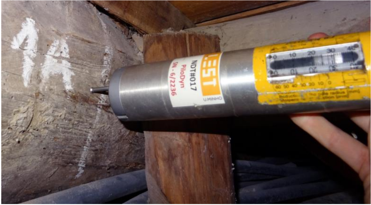
Figure 18 – Dynamic indenter Pilodyn® 6J Forest used for the Impact Penetration tests.
