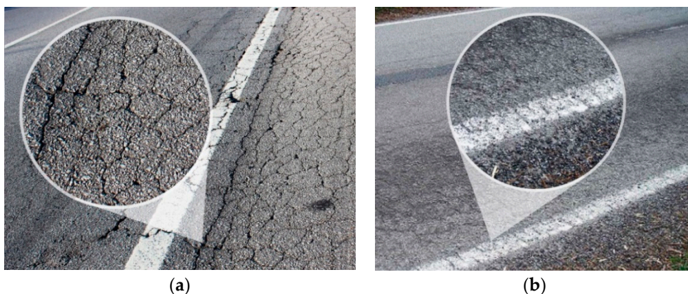
Figure 3. Examples of the distresses: (a) alligator cracking (ACR) and (b) raveling (R).
