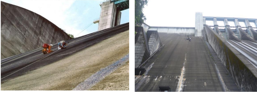
Figure 1: (Left photo) Climbing survey, (Right photo) UAV.
