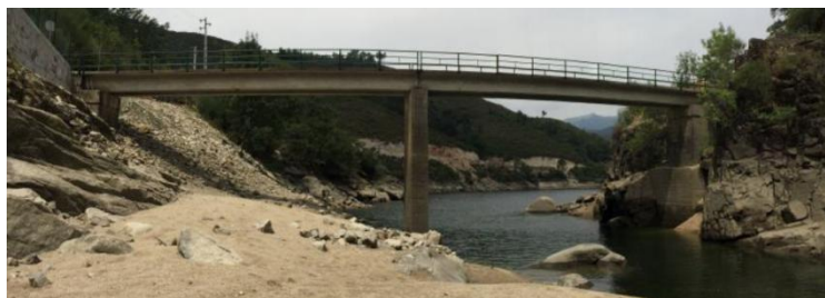
Figure 1: Overall view of Saltadouro Bridge (left side: North abutment; right side: South abutment).
