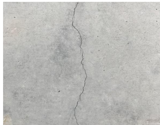
Figure 7: Surface cracking.
