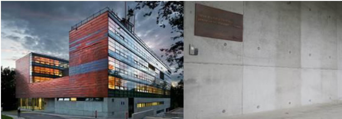
Figure 3: Photos of the entrance of Institute for Nanomaterials at TUL consisting of concrete panels which were protected by the BALCLEAN coating. To observe the self-cleaning function, only each second stream was coated, as illustrated in the picture on the right.
