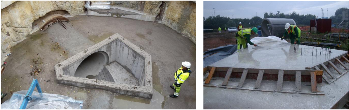
Figure 3: Inspection pit (left) and roof plate made of self-healing concrete with MUC+ (right)
