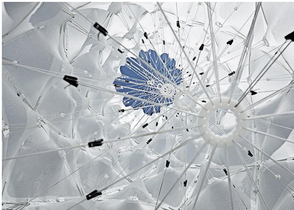
Figure 39, illustrates different components in a typical FRP rods structure with a fabric cover. (Corboy, 2017)
