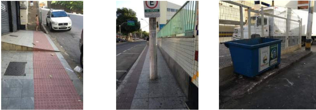
Figure 6: Incorrect execution of citizen sidewalk pattern and location of inadequate public spaces fixtures.
