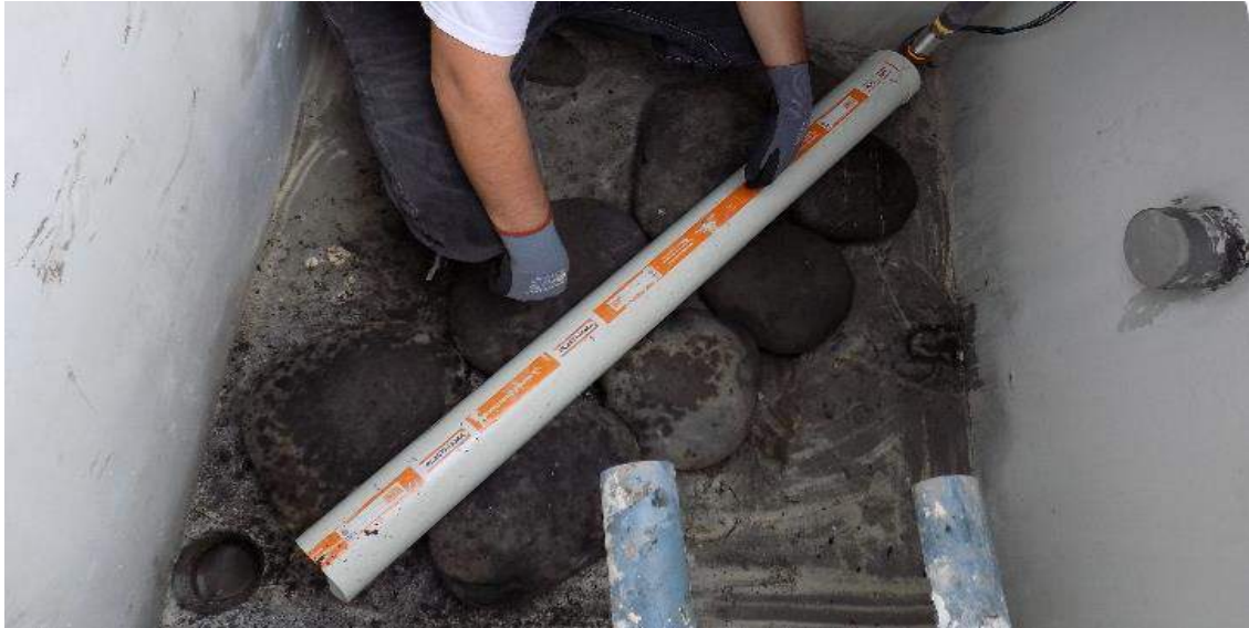
Figure 2. Installation of the submersible pump
