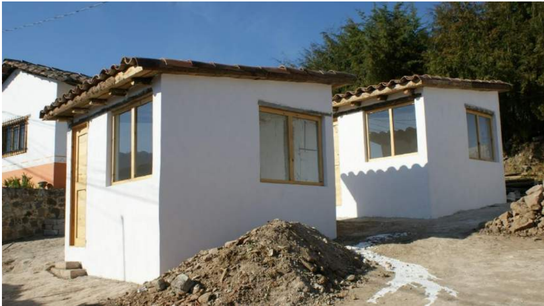
Figure 13. View of the two prototypes completed
