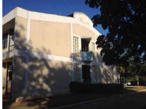
Figure 2 .West façade. Source: Authors,2015
