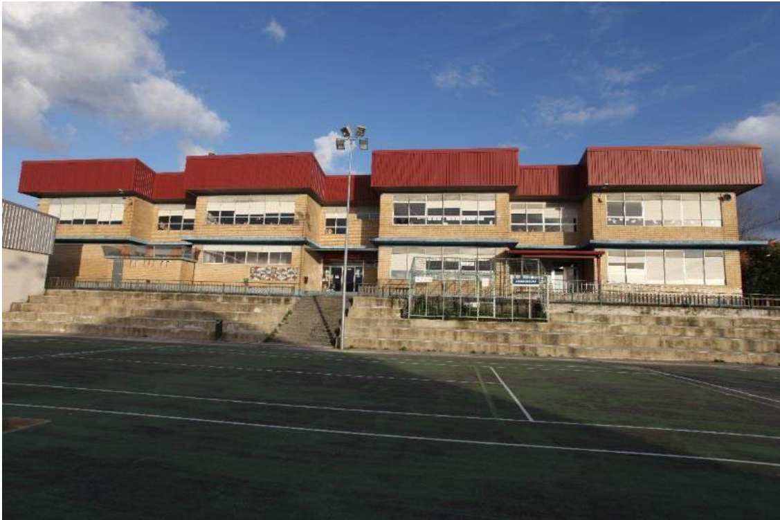
Figure 1. Study case. San Roque Elementary school in Cangas, Pontevedra, Galicia, España. West facade.
