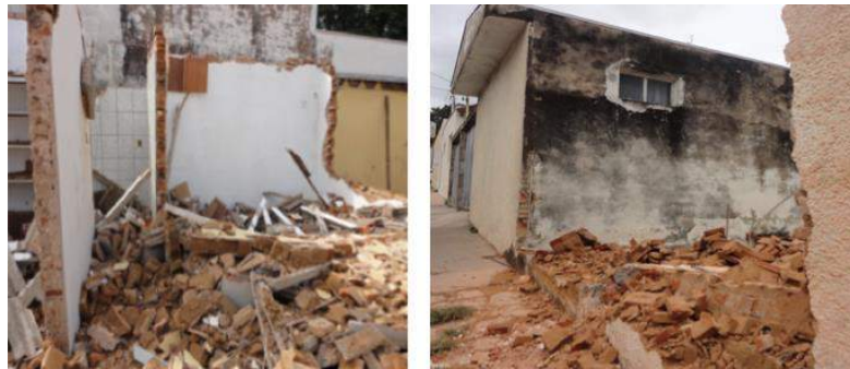
Figure 7 and Figure 8. Demolition of the internal and external walls. Source: Author, 2015
