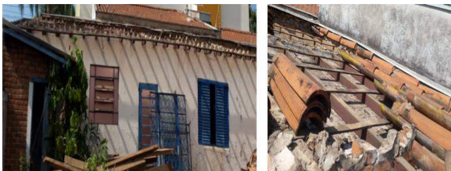
Figure 9 and Figure 10. Removing the coverage of the building. Source: Author, 2015
