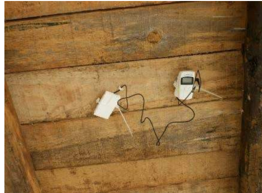
Figure 15. View of data logger to temperatures measure on the timber ceiling
