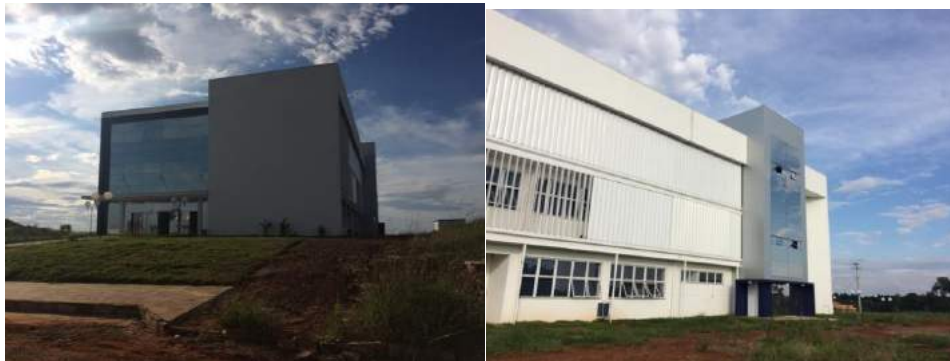
Figure 2. Building V2. South and East Façades.
