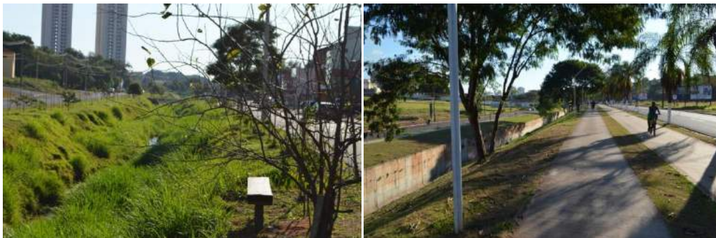
Figure 5. Alfredo Maffei Avenue in the first and second section, respectively.
