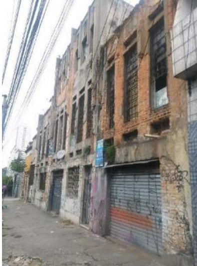
Figure 2 - Obsolete buildings (Celso Garcia Avenue)
