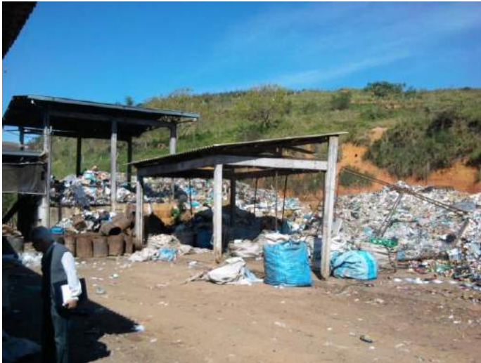
Figure 2 – Evidence of big amount of raw materials built up in the SCP's courtyard.
