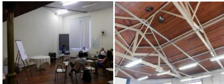
Figure 6: Teacher training centre, sign language class, opening on the second floor to the air vents. Air conditioning is provided in the reconstruction of the building.
