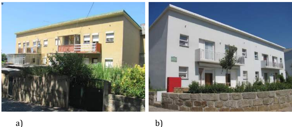
Figure 1 General aspect of the buildings a) before the intervention and b) after the intervention
