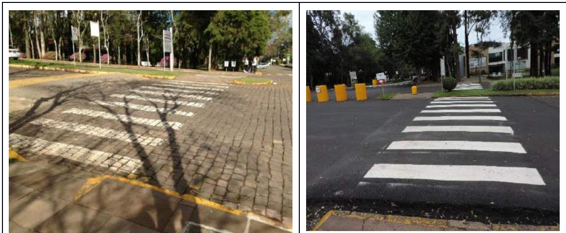
Figure 6. Raised sidewalk before and after modifications. Source: Authors, 2015.
