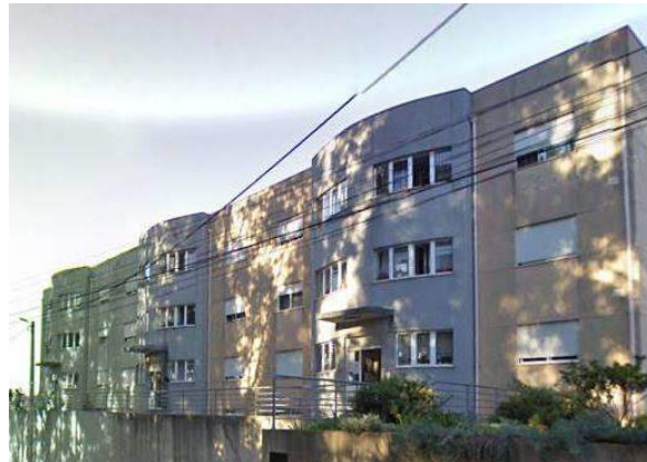
Figure 1 - Main façade of the building.
