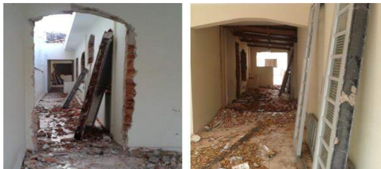
Figure 3 and Figure 4. Reuse of doors and windows. Source: Author, 2014
