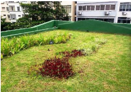
Figure 3: Green roof, Source: Author, 2016
