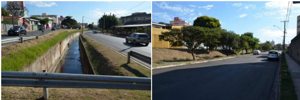
Figure 6. Trabalhador São Carlense Avenue in the unbuffered section
