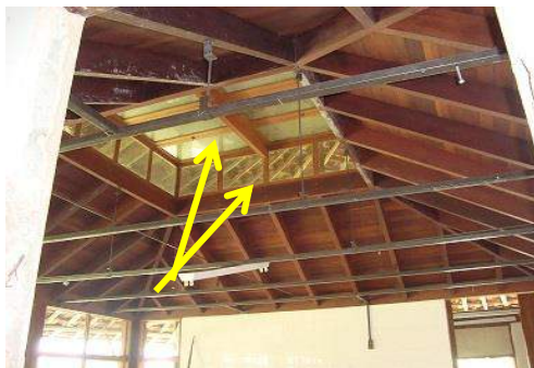
Photo 9 – Double protection and zenith ventilation
