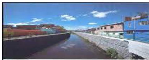
Figure 2: Situation after the removal of families. The stream resumed its original natural conditions and the families - without a housing alternative – moved to other locations not suited for urbanization. (Source: FONSECA; LUZ; CORREIA, 2014)
