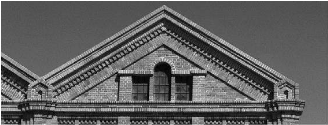
Figure 10 - Iconic historical building. Source – Author’s image.
