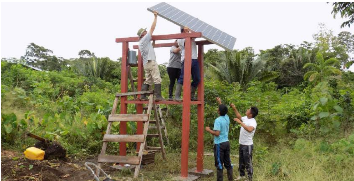
Figure 3. PV panel installation
