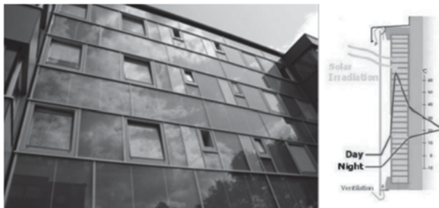
Figure 3. An indirect solar-comb construction BISTS.
