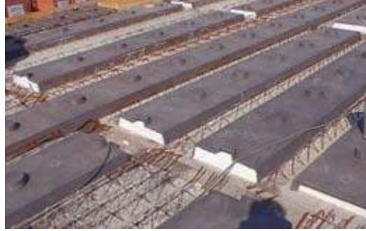
Figure 6. Installation elements from recycled plastic
