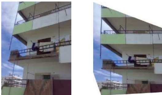
Figure 6. Shows an original photo on the left and a rectified one to the right.
