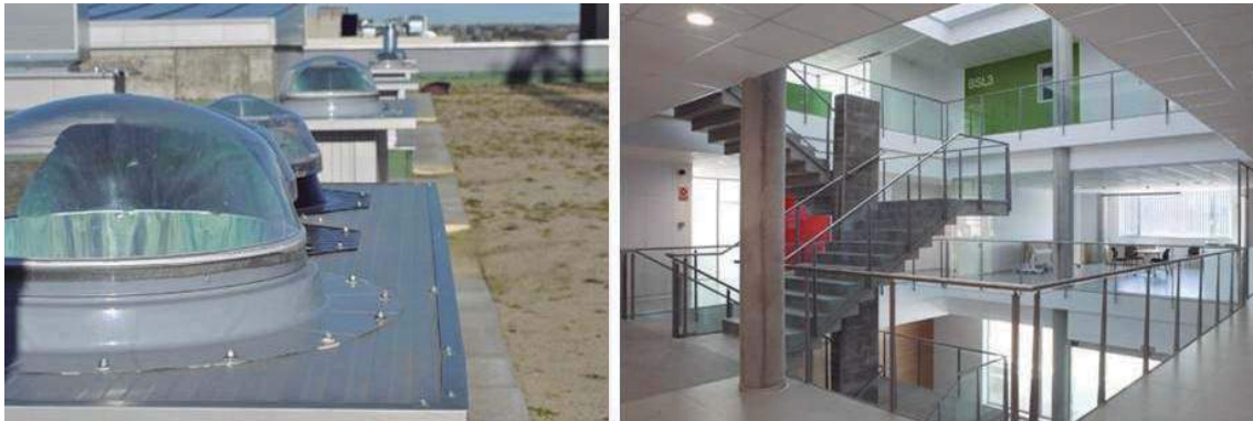
Figure 2 - Tubular day lighting devices (Solatube) on the green roof and the internal skylight above staircases.
