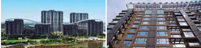
Figure 4. View of the building complex and of the system (Global Solar Thermal Council, 2014; Renewable World, 2014)
