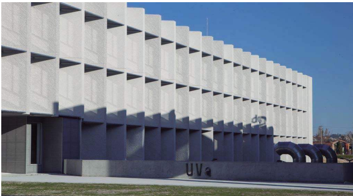
Figure 11. LUCIA building. North-West façade and geothermal tubes.
