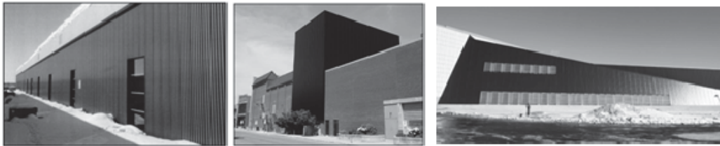
(a) Canadair facility (b) Avon theatre, Canada (c) Toronto airport, Canada Figure 5. Applications of transpired air collector in various buildings.
