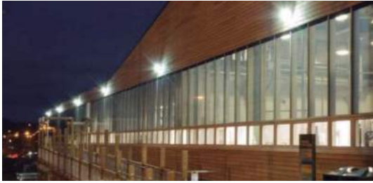
Figure 7. View of northern facade consisting of photovoltaic glazing ( Mc Ildowie, 2014).
