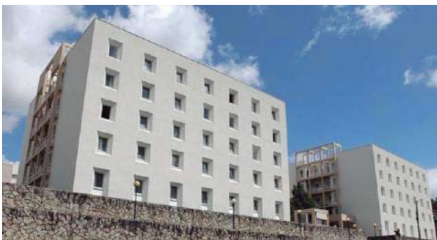
Figure 4. Photo of the case study buildings complex (Serviços Acção Social, 2014).
