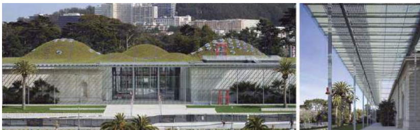
Figure 6. View of the Academy and the circumferential canopy with the photovoltaic cells (California Academy of Sciences, 2014;DeZeen Magazine, 2014).
