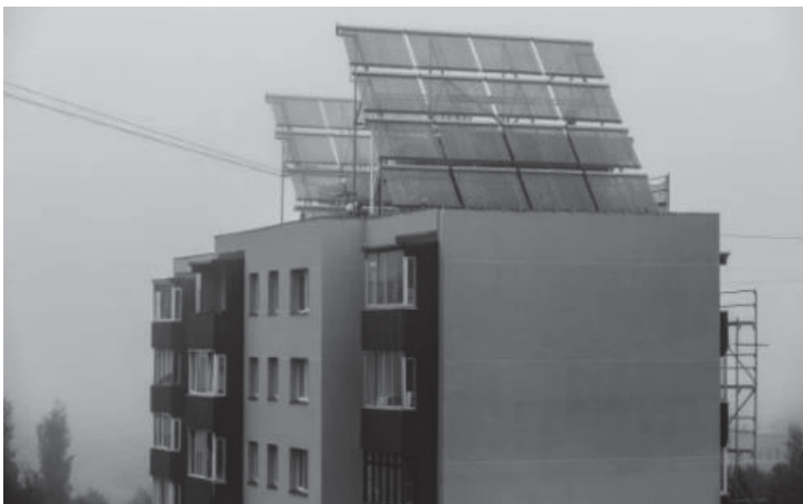
Figure 1. The view of the house with the solar thermal system.
