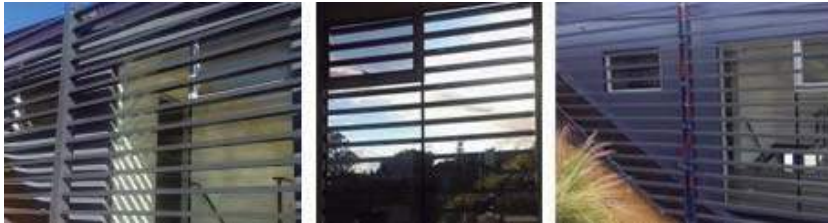
Figure 2. Examples of the Unglazed Flat Plate Hydraulic Collectors with visible pipes (BioTecture, 2014)
