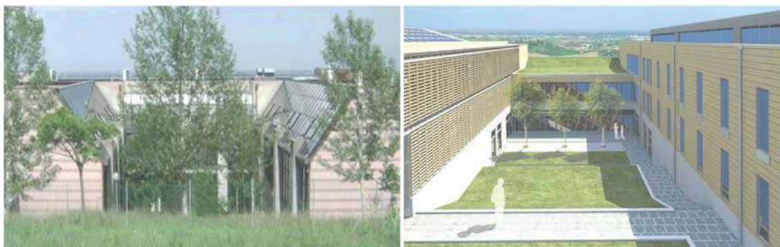
Figure 3. The pictures shows the result of a study about the potential impacts of a school renovation. The main improvements deal with the energy performances, indoor and outdoor quality, comfort conditions.
