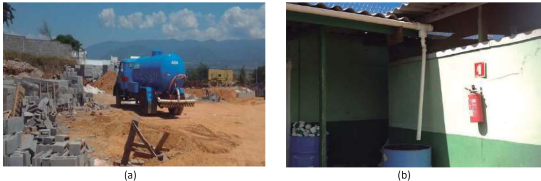
Figure 2 - Sustainable Practices Site B (a) Water tanker vehicle to irrigate construction site (b) Collection of rainwater by the roof
