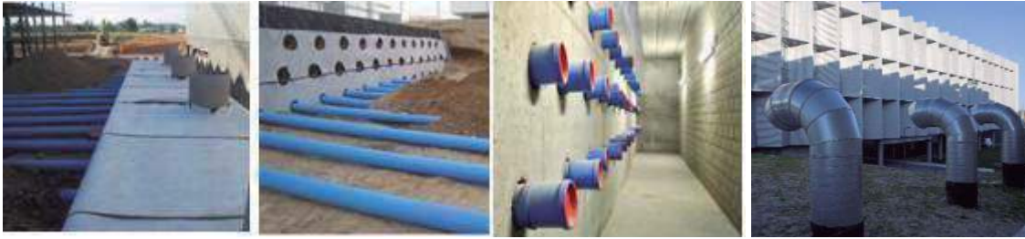
Figure 5. Different construction phases of geothermal pipes.
