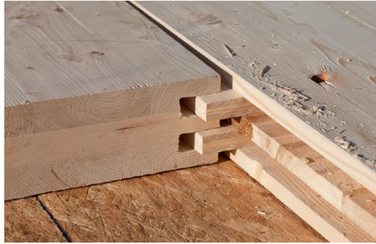
Figura 4.22 – Double internal spline.
