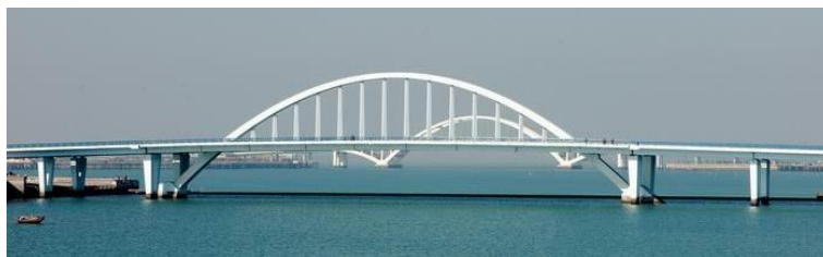
Figure 1 : Tianyuan Bridge (behind is Wuyuan Bridge)
