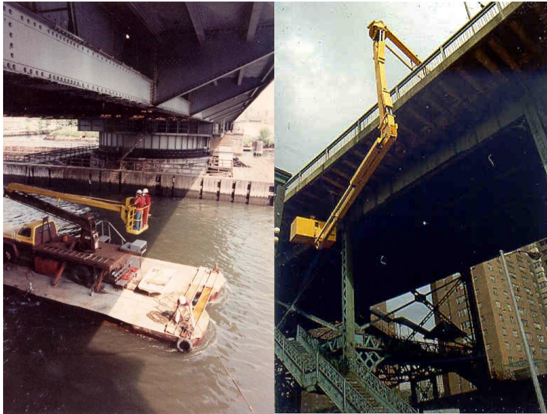
Manual inspection using a movable inspection gondola
