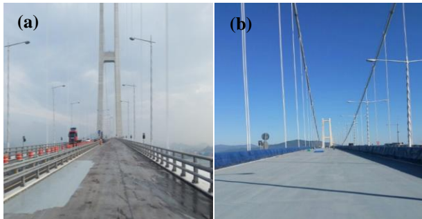
Fig. 10. Guardrails on decks (a): As-built, (b): Covered by temporal screens
