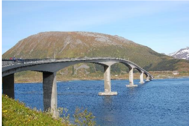
Fig 1. The Gimsøystraumen bridge in Northern Norway (Lofoten area)
