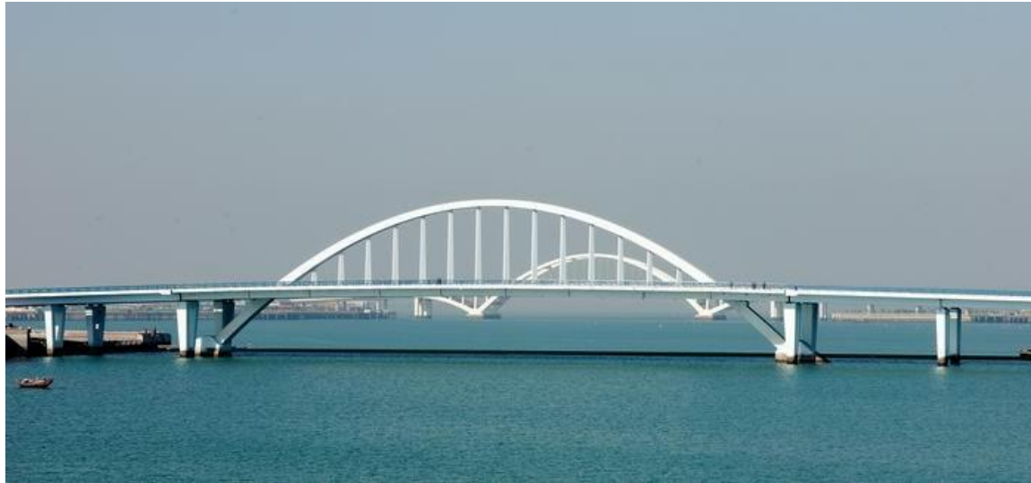
Tianyuan Bridge (behind is Wuyuan Bridge)
